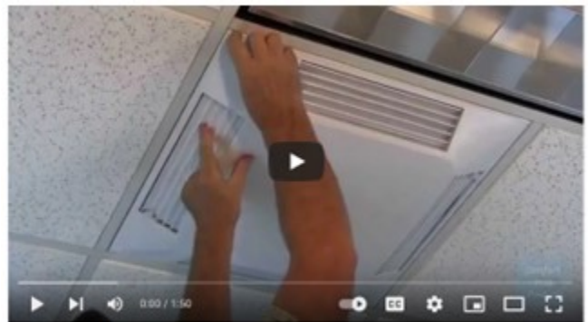
Comfort First Introduction and Installation
